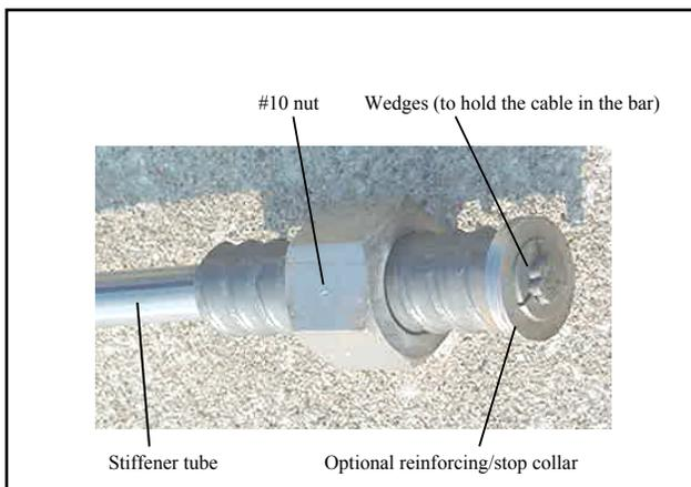
Figure 5 – Detail of the tensioning mechanism
