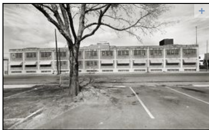
The Walter Tips Co. Warehouse, 215 W. Second St., looking north in 1982. The warehouse was razed in 1985 and Amli ... Read More
