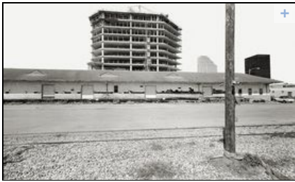
Republic Square One, now the Hobby Building, 333 Guadalupe St., under construction, looking northeast from West Second Street in 1984.
