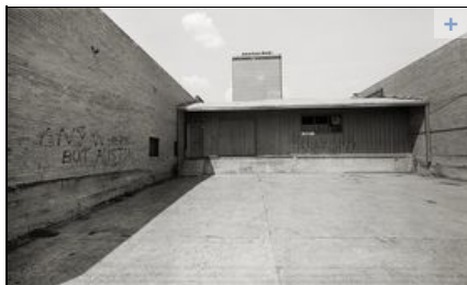
Alley behind the 200 block of West Fourth Street, looking north toward the American Bank Tower in 1982.
