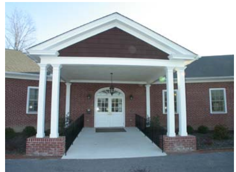
private entrance w/ handicap accessibility
